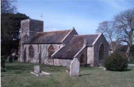
The cracking in the walls was mostly due to the vaulted ceiling structure allowing too much spread onto the walls thus creating cracking against the existing tower walls and the Chancel arch which was erected first. There were further cracks associated with the later addition in the 1880's of the Vestry on the south side of the Chancel.
